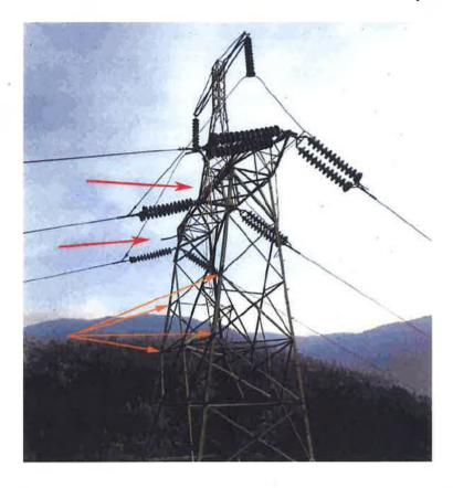
Tower :27/222's jumper extension broke and allowed the uninsulated transposition jumper to dangle free and contact the jumper arm extension. The following enlargement from the photograph of the similar, undamaged tower shows where the attachment of the suspension insulator to the jumper arm extension failed.
